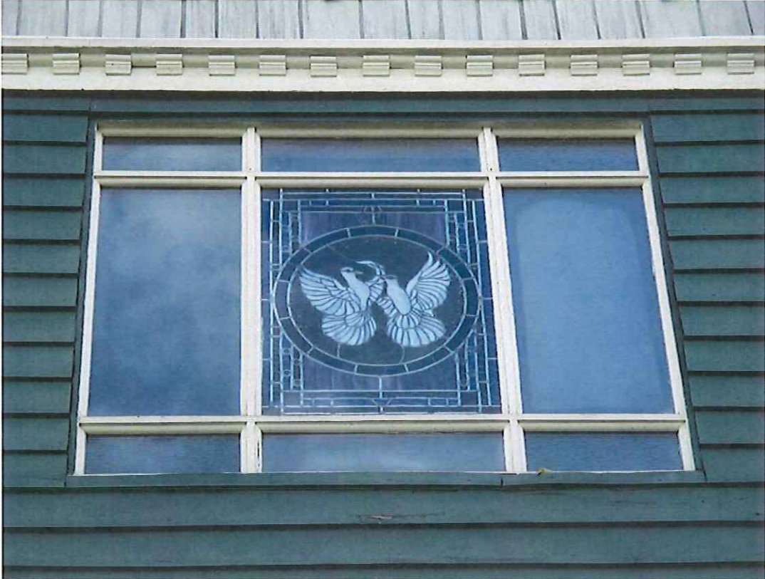
Below: current detail view of large modern window to be replaced with wood double hung window
